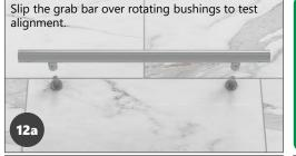
**Pro Tip** After confirming alignment, take a permanent marker and draw a line across the top length of each rotating bushing (both inner and outer components). Securely torque the 10-24 screws using a #2 Phillips (only use a hand screwdriver). The objective is to keep the lines from separating as you tighten.
